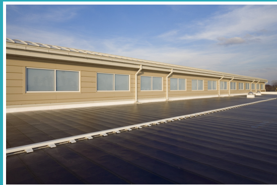
(Right) Daylighted Classroom and (Left) Rooftop Thin Film and Crystalline PV Panels Source: Rachel Paul Photography (for CMTA Engineers)
