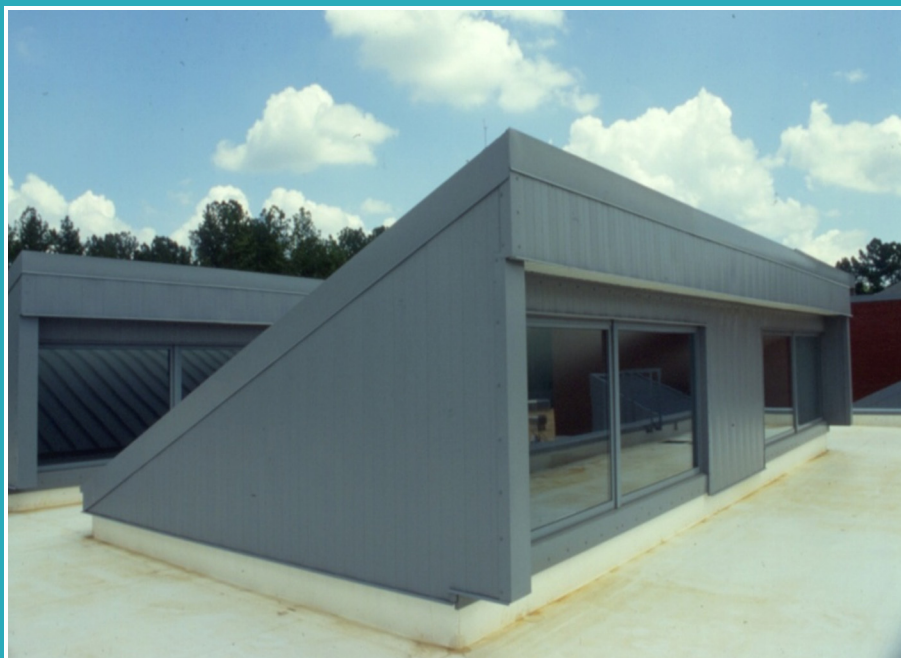
South-Facing Roof Monitor
