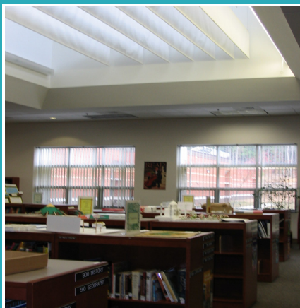
Libraries/Media Centers Using South-Facing Roof Monitors with Baffles
