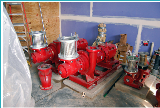
Pump for Closed Loop Hybrid Heat Pump System Source: Greensburg GreensTown (courtesy of DOE/NREL)
